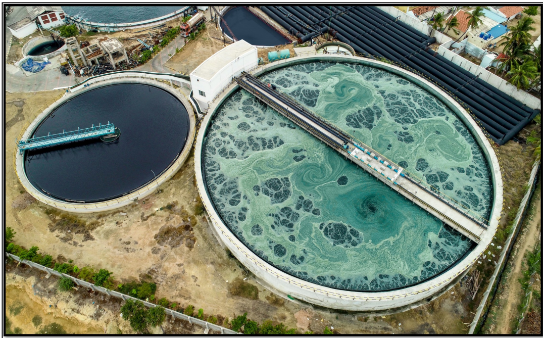
AERATION TANK & SECONDARY CLARIFIER
