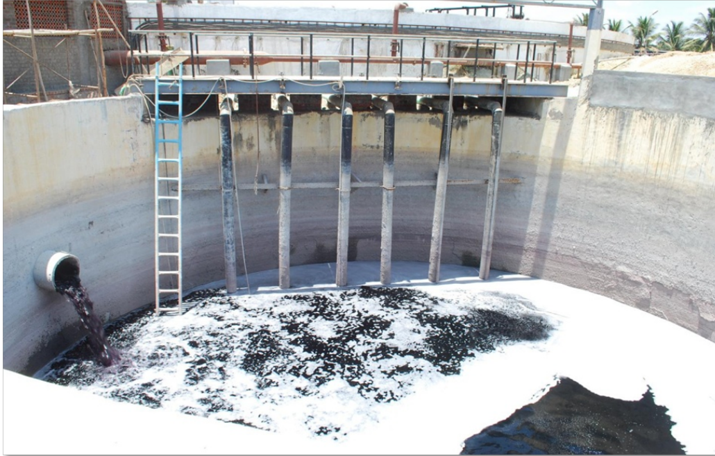
RAW EFFLUENT RECEIVING SUMP
